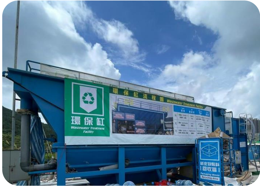
Three wastewater treatment facilities are setup on site to treat the wastewater generated on site.
