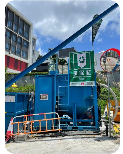
Three wastewater treatment facilities are setup on site to treat the wastewater generated on site.
