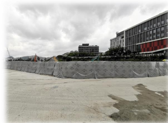
Setup temporary noise barrier
