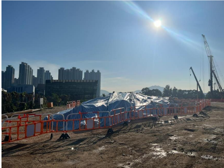
Open stockpiles of construction materials or exposed slope surface are covered by tarpaulin.
