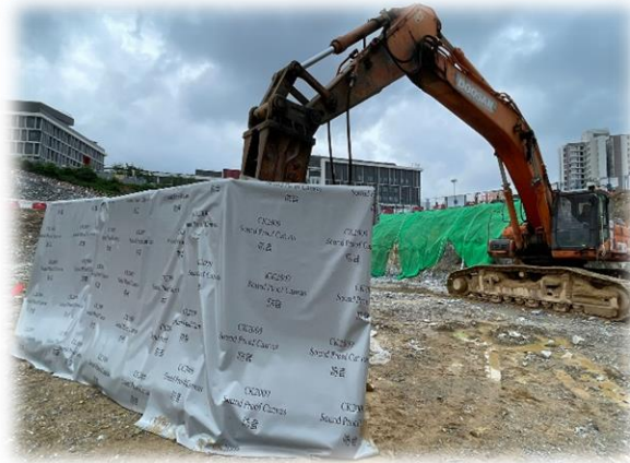
Setup movable noise barrier
