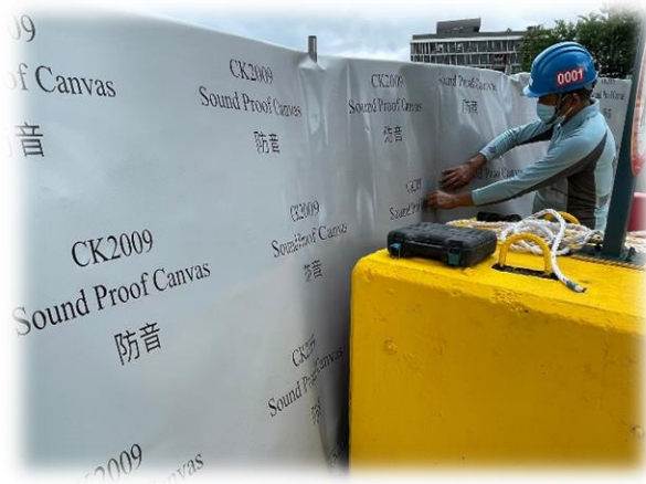
Setup temporary noise barrier
