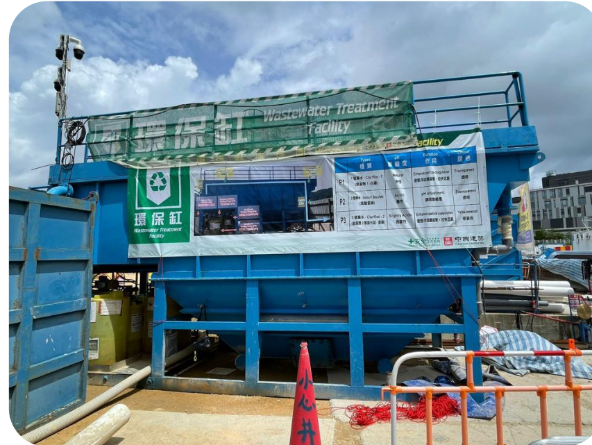
Three wastewater treatment facilities are setup on site to treat the wastewater generated on site.
