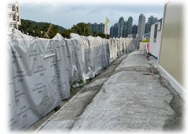
Setup noise barrier at site boundary
